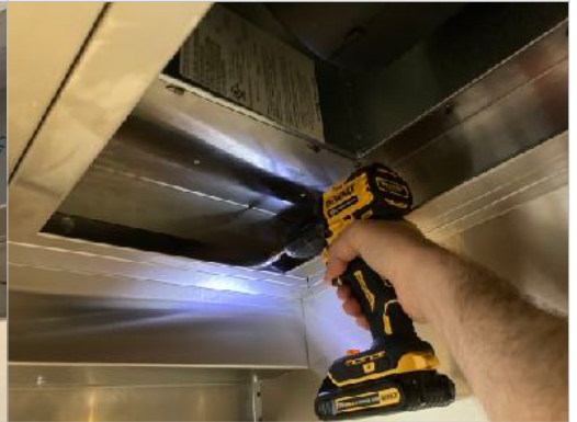
24. Install Motor / Blower Insert flush to the underside of the hood mounting flange using SS self-tapping screws.
