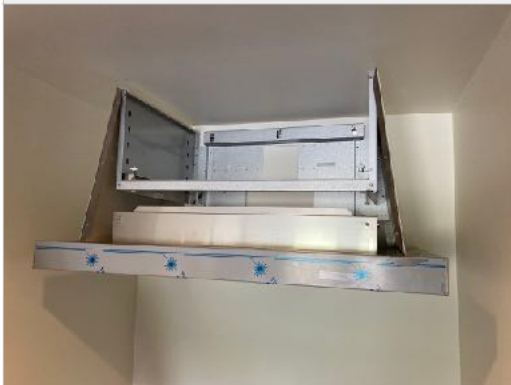
16. Hang hood body centered on support bracket and level unit using the [2] M5 x 40 leveling screws.
