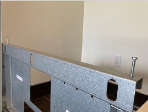
14. Insert the [2] M5 x 40 leveling screws into the threads on top of the hood body rear panel.
