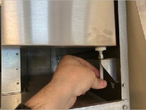
26. Install and raise the duct cover against ceiling / soffit surface and if clearance allows, secure with appropriate screws into place.
