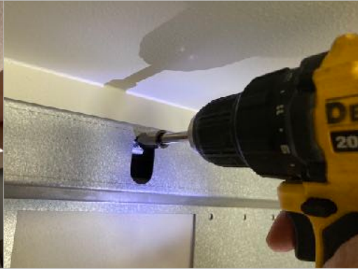
20. Once level, secure the hood to the wall by fully tightening the M6 x 30 screws. This pulls the rear panel to the wall.
