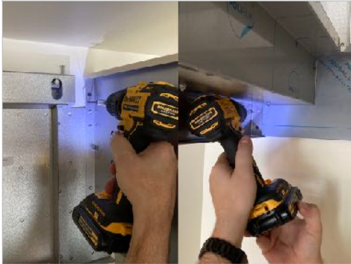
22. It is imperative to secure the upper and lower hood body corners to the wall with the appropriate screws. Use both mounting holes provided.
