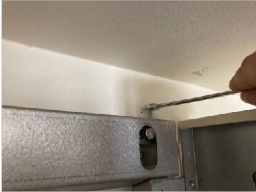
19. Level the hood body by tightening or loosening the [2] left or right M5 x 40 screws.
