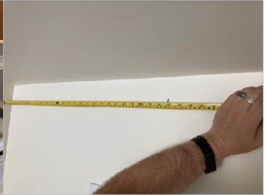
12. Measure and mark the mounted hood body centerline at the support bracket mounting location.
