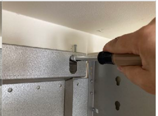
18. Hand tighten the M6 x 30 screws lightly to flatten the hood body to the wall but to still allow movement.
