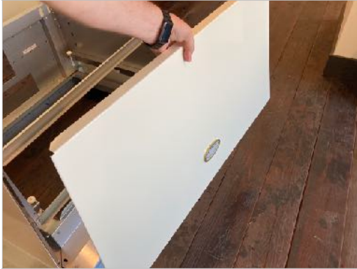
10. Carefully remove hood body front panel towards the front and set aside.
