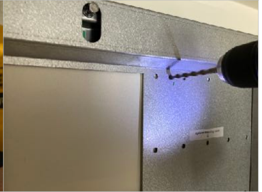
21. Screw rear body panel to wall into studs were possible near the top and bottom of the rear panel. Drill new holes through panel as needed to align to studs.
