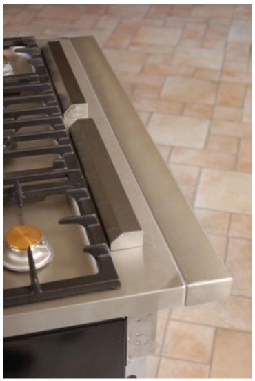
Since the height of the range is adjustable, the spacer should be able to slide just under the backsplash material at the exact height of the counter surface (fig.A). **Do not grout or cement** the spacer into place! The range must retain the ability to pull away from the wall for future service needs.
