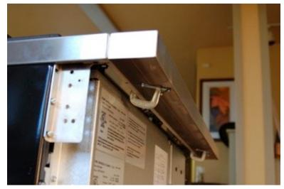
The island back Spacer must be used with a noncombustible flame-retardant backsplash material (tile, metal, stone, etc.) installed on the wall above the cooking surface.
