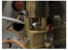
2. Now adjust the air collar for each burner. Standard sea level adjustments are as follows: [5k btu = 1mm open\*], [11k btu = 1/2 open], [15k btu = Max open], [18k btu = 3/4" open] -Now adjust the low flame height for each burner by adjustment of this needle valve screw.
