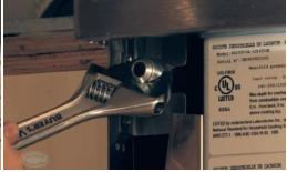
Now connect the flex line to the compression fittings. The compression fittings do not require compound sealant, but must be made tight enough to prevent fuel leakage. Use a wrench on each hex fitting to ensure tight seal.
