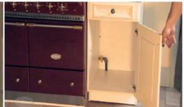
After the fuel line is installed, open the gas cut-off valve and check for leaks with bubble fluid at every connection joint. Close the gas valve and refit any joint that has bubbles form.
