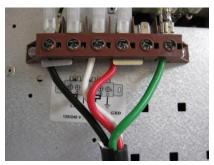
1. Check the terminal block connections. Make sure all terminal screws and jumper bars are in place and tightened.
