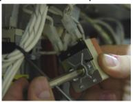
4. As a general rule, the amount of rotation applied to the collar is equal to the rotational difference between the <u>actual</u> average oven temperature and the <u>target</u> average temperature as seen on the oven dial. (i.e. the temp difference on the dial is the collar adjustment difference.)
