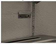
Push the range into position as close to the wall as possible. Adjust the range feet to level and bring the range height to the desired level. Measure 4" up from the steel range top and make a mark on the wall on each side of the range. Draw a straight line between both marks using a string or ruler. Install each bracket by lining up the center of the screw holes on this line. Run the screws directly on the line, use wallboard anchors if necessary.
