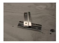
Position these brackets on the wall evenly behind the range making sure one bracket is at each corner. Install each bracket with the screw holes facing down and the hook ledge away from the wall.
