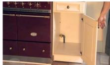
After the fuel line is installed, open the gas cut-off valve and check for leaks with bubble fluid at every connection joint. Close the gas valve and refit any joint that has bubbles form.
